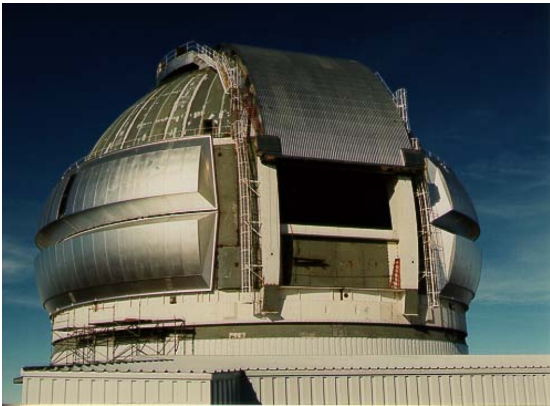
The Mauna Kea enclosure showing the vent and shutter, late October 1997.
