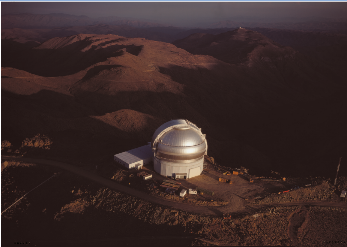
Aerial photo of Gemini South - April 2000
