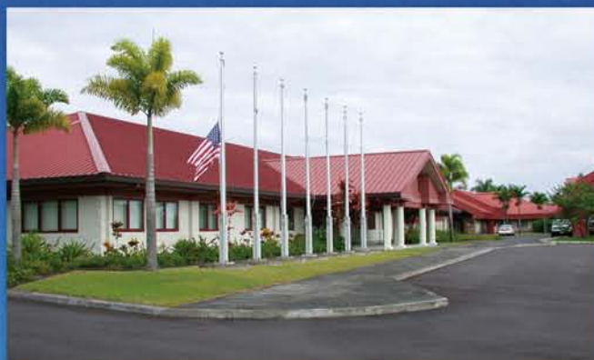
Gemini Base Facility September 11, 2001
