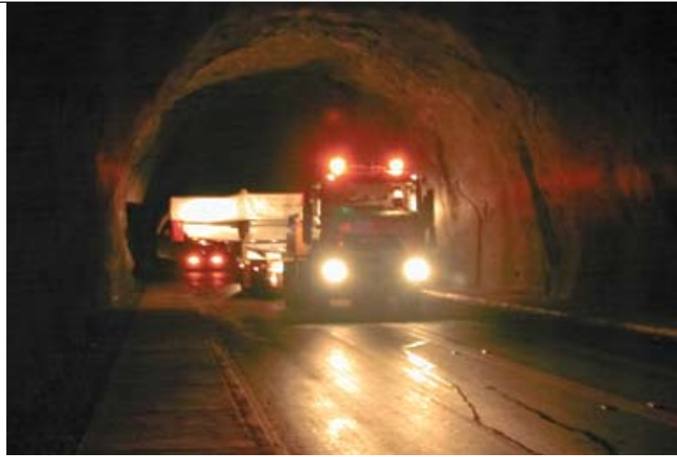
Figure 4. The Gemini South mirror being transported through the Puclaro Dam Tunnel which was enlarged from its original 8-meter width to 10 meters to accommodate the Gemini loads to Cerro Pachón.
