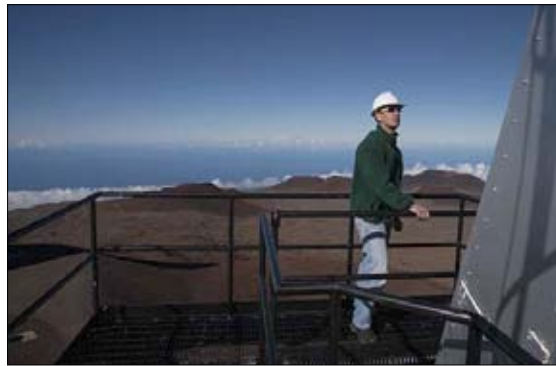
Figure 2. View from the newly installed Shutter Service Platform at Gemini North, installed to facilitate safety and accessibility during shutter motor servicing.
