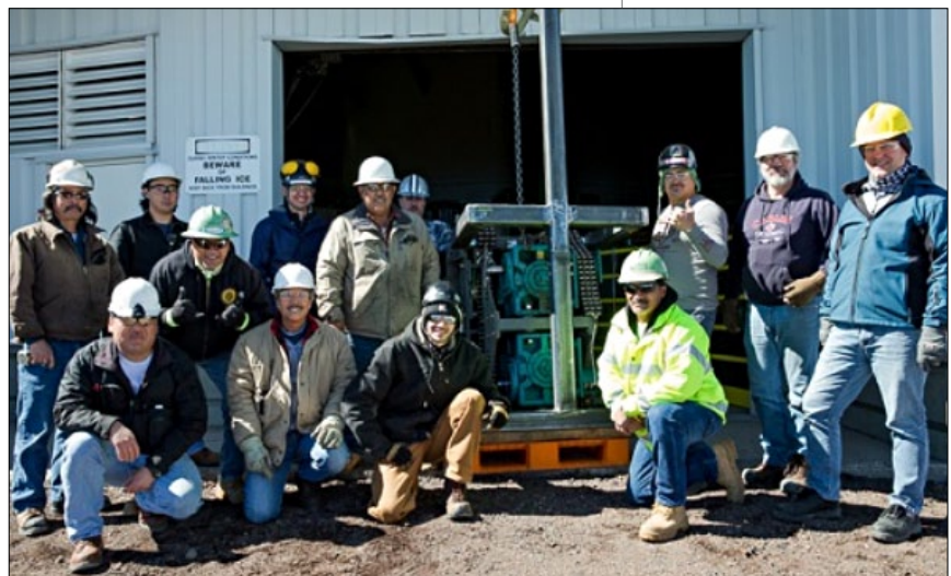
Figure 12. The dome repair team, just before lifting the repaired gearbox back into position.
