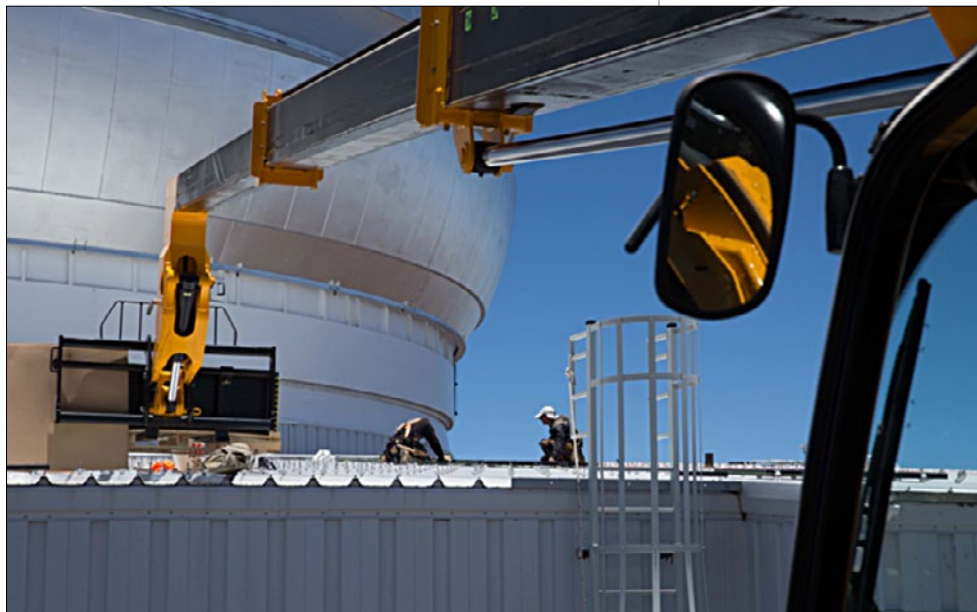
Figure 1. The PV panels were transported to the roof by crane.
