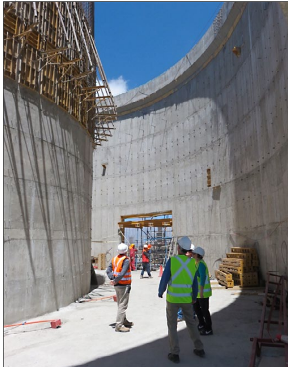
Figure 2. Staff and visitors inspect the LSST pier and enclosure.
