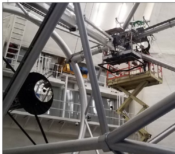
Figure 10. Installing GNEST onto telescope truss below top ring. Credit: All photos this page by Jeff Donahue
