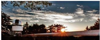
Figure 2: The E2 telescope and the start of the 150-meter vacuum pipe that conducts the light beam to the combining area. *Credit: S. Golden/Georgia State University*
