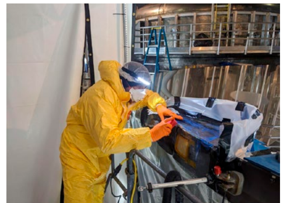
Figure 4: Thierry Lagrange grinding of Damage Area #1. Credit: Safran-Reosc
