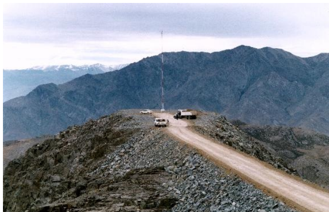
Figure 1. The SOAR site, looking northwards (into the prevailing wind) from below the Gemini-South enclosure. The terrain drops off for thousands of feet on the NE through W sides of the site, and for several hundred feet on the E side. Site leveling had been completed at this time and the dump truck was laying down a thin cap of dirt.
