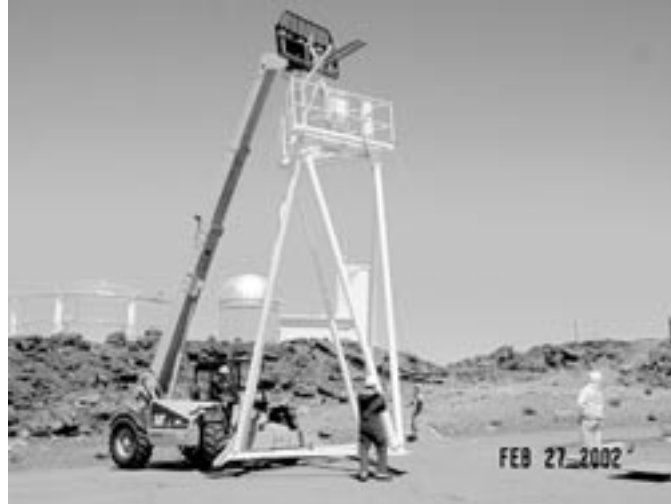
Installing the test stand at Haleakala.
