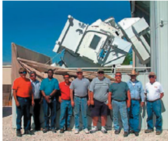
The SOLIS VSM instrument installed on the mount at the GONG farm temporary site, with the installation team, from left to right: Kenny Smith (Mid-States Co.), Benny Bracamonte (Marco Co.), James Robinson, Sean Hofhine (Mid-States Co.), George Luis, Dave Jaksha, Dave Hauth, Neill Mills, and Lou Lederer.
