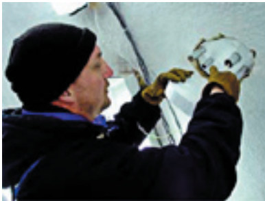
Figure 2. Dave Hauth (NOAO) installing sensors at Gemini North for ATST.
