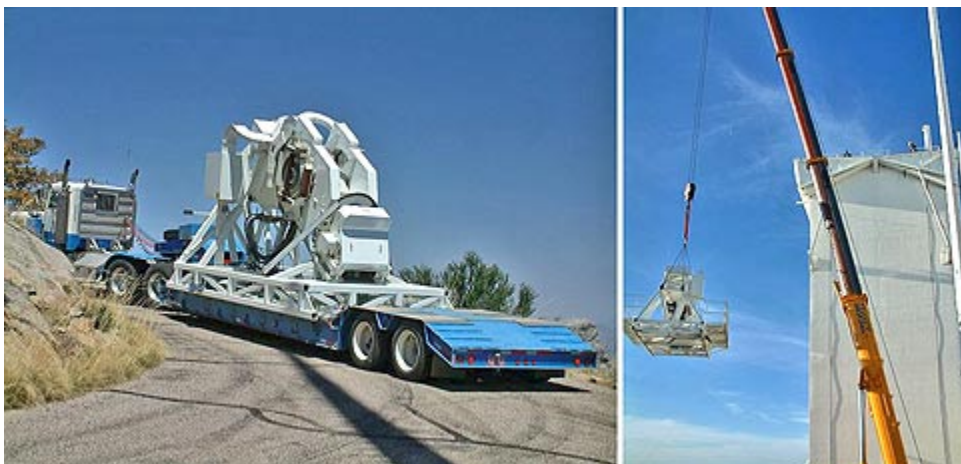
Figure 1. The SOLIS mount arrived on Kitt Peak and was lifted to the top of the old Vacuum Telescope tower in April. (Photographs by David Jaksha.)
