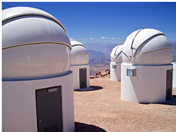
Four of the six PROMPT enclosures have already received 12-foot diameter clamshell domes built by Astro Haven. The remaining two enclosures will receive domes in September 2005. Live images of PROMPT can be viewed at www.physics.unc.edu/~evans/promptcam/promptcam.html .
