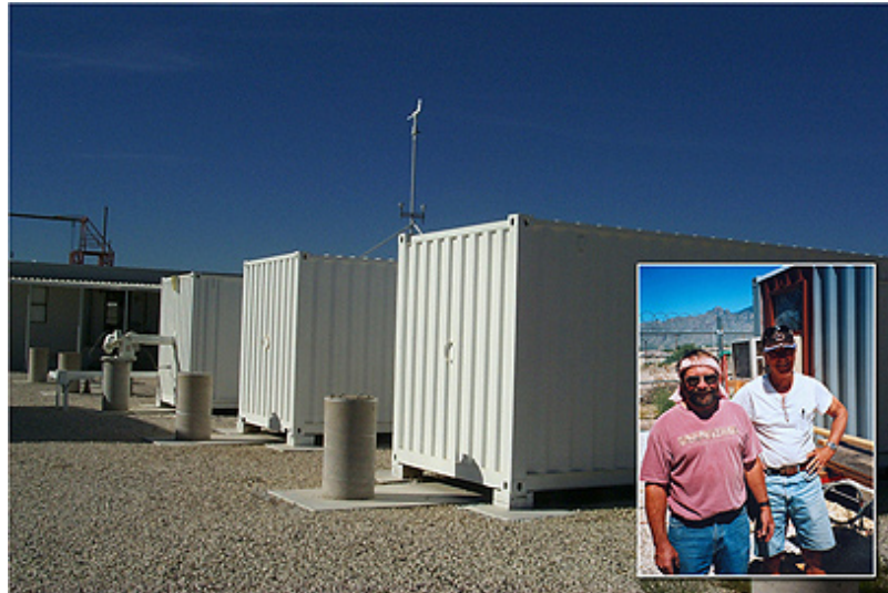
Figure 2. Last summer, two shipping containers were delivered to the GONG Farm. Now, a little more than six months later, thanks to Terry Bender and Jim Mason (shown in the inset photo) and the rest of the team, the new GONG shelters are ready to go. One was shipped to Australia in February to replace the one that's rusting away. The swap is scheduled to begin in May 2006. The other one will house GONG's "hot spare." The hot spare project is currently ramping up and is scheduled to be complete by the end of FY 2007.
