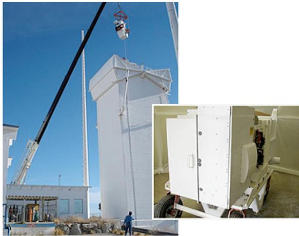
Figure 1. The Vector Spectromagnetograph (VSM) instrument weighs approximately 3,300 pounds, and must be lifted roughly 75 feet to its mount on the SOLIS tower. Members of the SOLIS team and Kitt Peak National Observatory staff assist the crane operators to move the instrument safely and successfully. The inset image shows the VSM on a custom cart within the temporary clean area, where it resided for just over seven weeks during modulator replacement, grating repair and camera tests.
