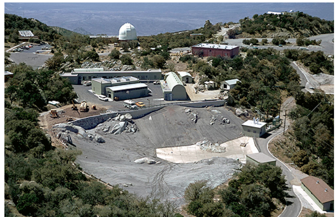
Figure 3: Kitt Peak water system rain catchment basin (without any water in it). (Photo credit: NOAO/AURA/NSF)
