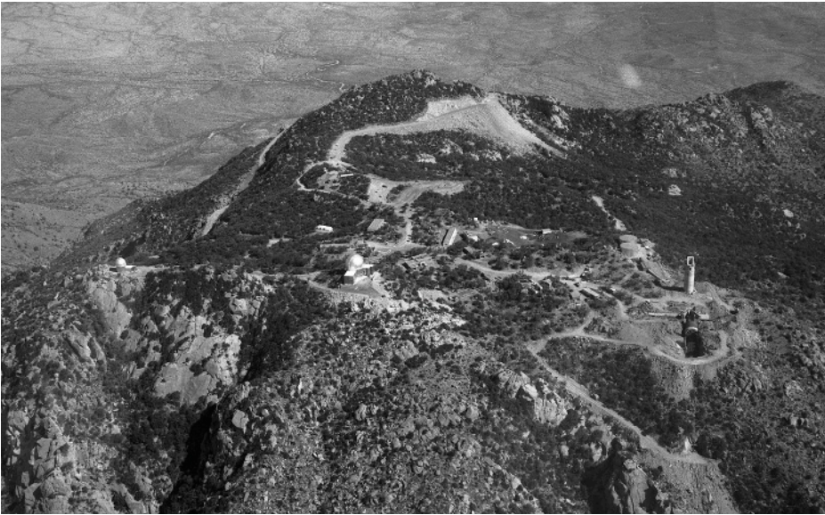
Figure 2: Kitt Peak in 1961 had completed domes for 36-inch (0.9-meter) and 84-inch (2.1-meter) telescopes and administration and maintenance buildings with construction of the Solar Vacuum Telescope underway.
