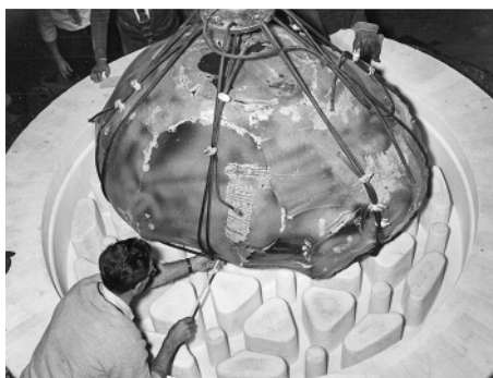
Figure 7: Loading of the raw glass for the 84-inch mirror into the furnace at Corning Glass.
