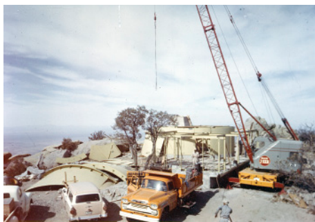
Figure 6: Early construction work on the dome for the first 36-inch telescope.
