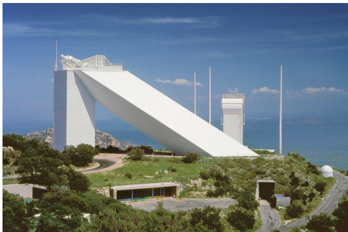
Figure 1: McMATH-Pierce solar telescope (foreground) and SOLIS Tower surrounded by three lightning protection towers (background) on Kitt Peak. (Image credit: NSO/AURA/NSF.)
