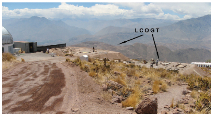
Las Cumbres Observatory Global Telescope Network construction work at Cerro Tololo has started. (Image credit: N. van der Blik.)
