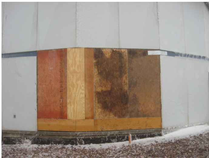
Storm damage and temporary repairs to WIYN 3.5-m telescope dome and support building. (Image credit: John Dunlop.)
