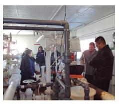
Figure 11: Kitt Peak pump house for the water distribution system. This facility will undergo a major renovation in FY12. The project has been developed and is out for bid to external contractors (some of whom are shown here reviewing the existing pumps, piping, and filters that will be replaced). The total project is valued at approximately \$1M. (Image credit: Kate Foster, NOAO/AURA/NSF.)
