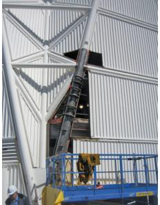
Figure 3: Repair of Mayall 4-m telescope column with strongbacks. (Image Credit: Kitt Peak Facilities, NOAO/AURA/NSF.)
