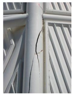
Figure1: Cracked column on Mayall 4-m telescope. (Image credit: Kitt Peak Facilities, NOAO/AURA/NSF.)
