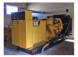
Figure 3: New backup generator for Cerro Tololo installed near the summit. (Image credit: Enrique Figueroa, NOAO/ AURA/NSF.)
