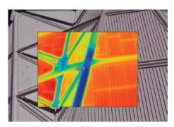
Figure 2: Thermal picture of the ice plug in cracked column. (Image credit: W. Goble, NOAO/AURA/NSF.)
